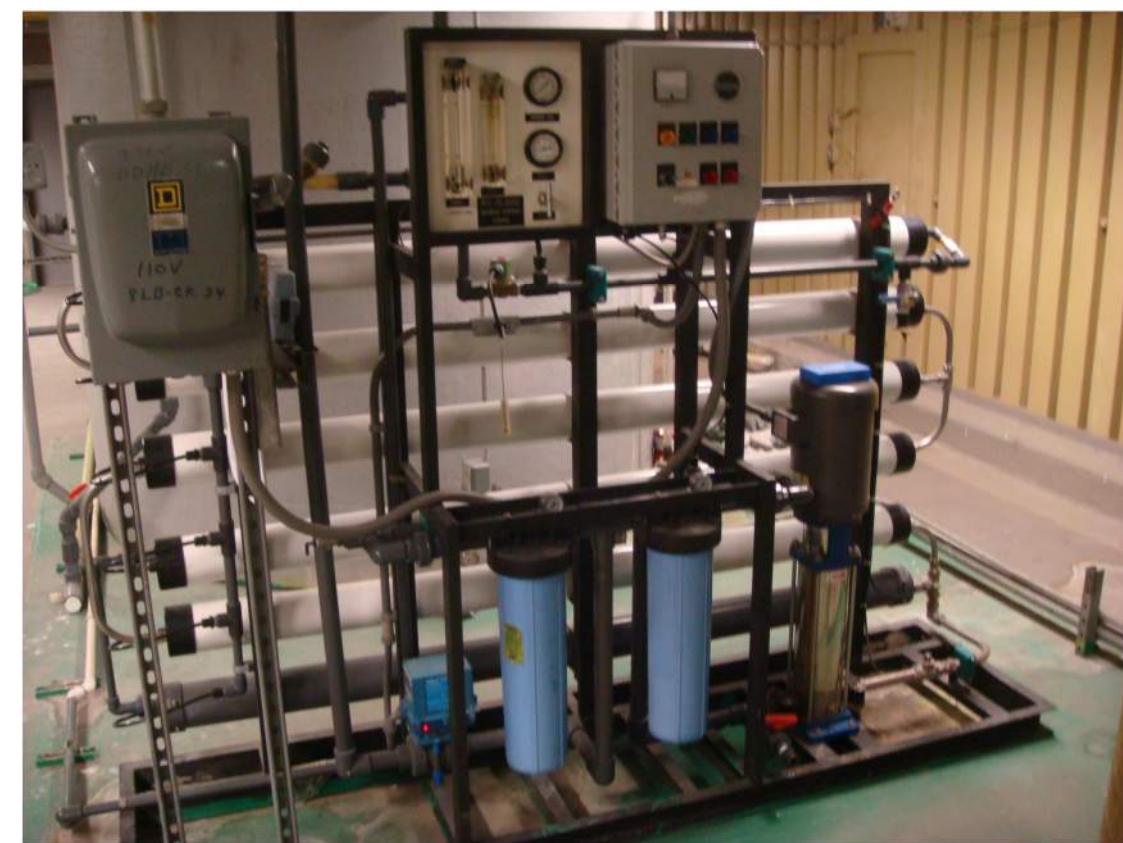
03 RO SYSTEM LOOKING NORTH NOT TO SCALE
