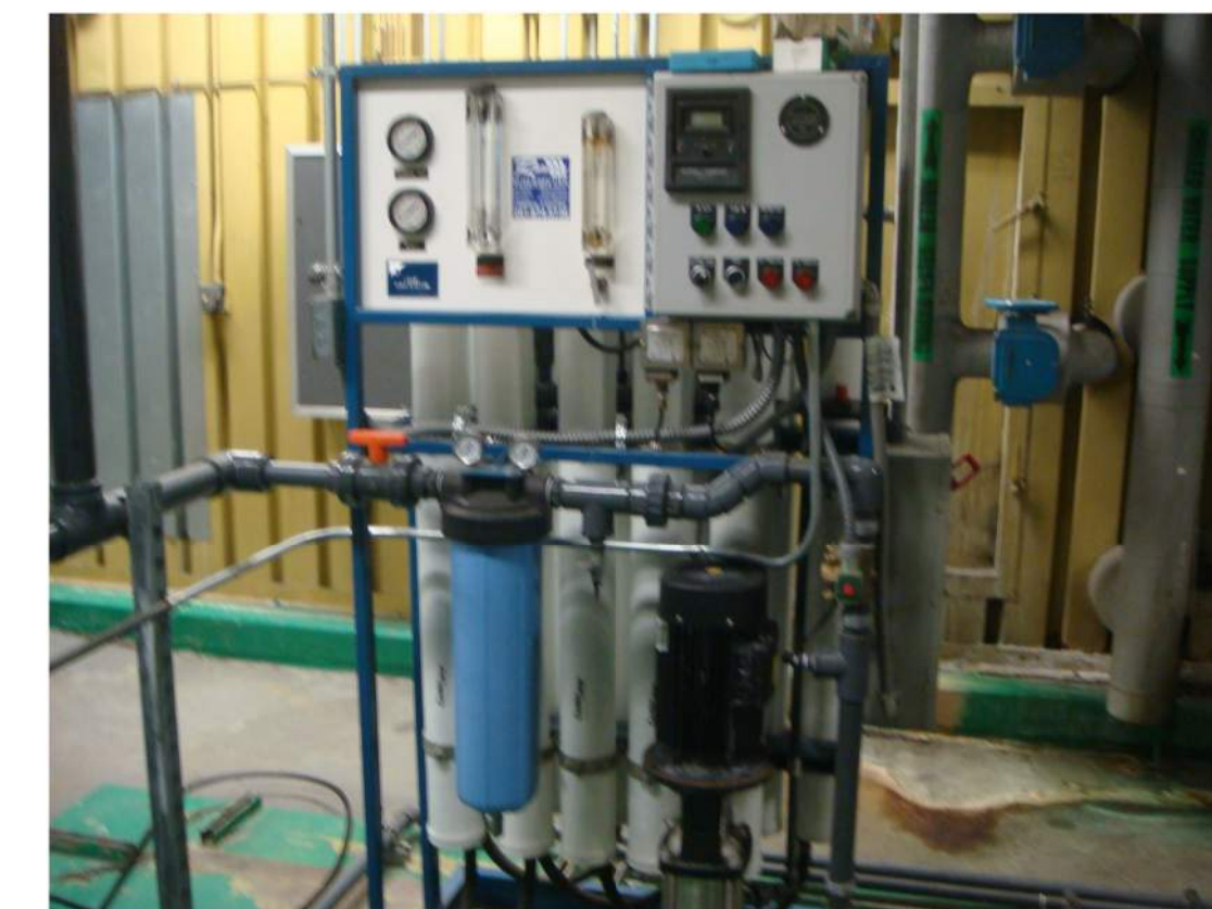
04 RO SYSTEM LOOKING EAST NOT TO SCALE
