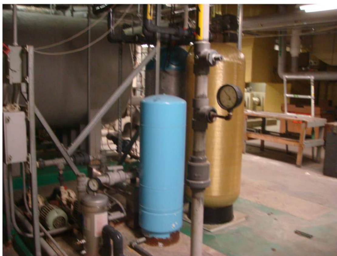
04 RO SYSTEM LOOKING SOUTH NOT TO SCALE
