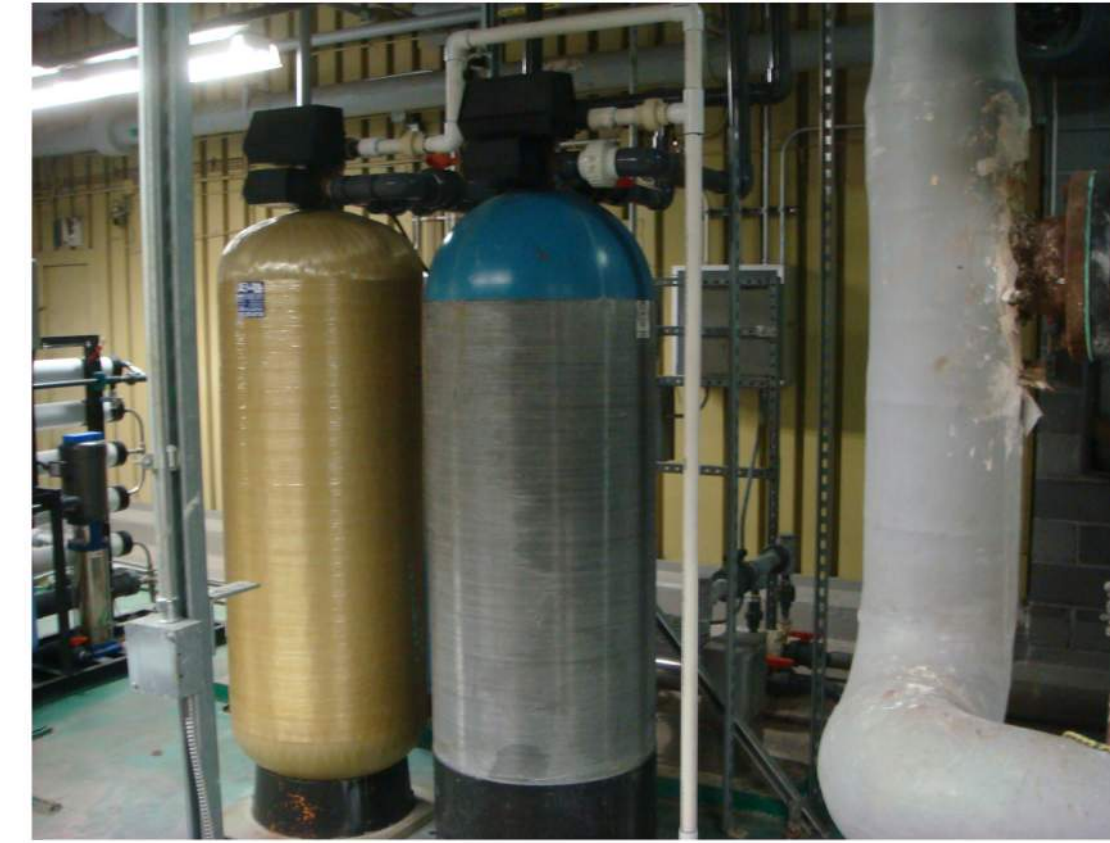
05 CARBON FILTERS LOOKING EAST NOT TO SCALE
